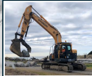
CATERPILLAR TRACKED EXCAVATOR EXCAVATING SAND AND PLACING ROCKS
