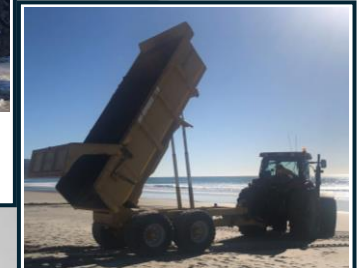
TRACTOR/TIPULATOR UNLOADS ROCKS DOWN 1.5m ONTO SAND. LOCATION VARIES WITH WORKS THROUGH THE DASHED AREA.
