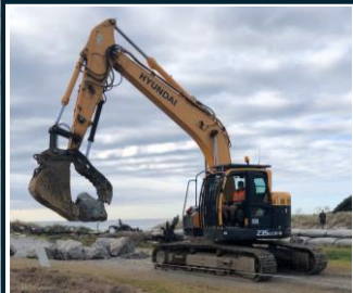
CATERPILLAR TRACKED EXCAVATORS MOVING ALONG CREEK PLACING ROCKS TO WALL
