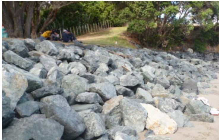
Photograph 3.5.2: Rock revetment at Matheson Bay, Auckland
