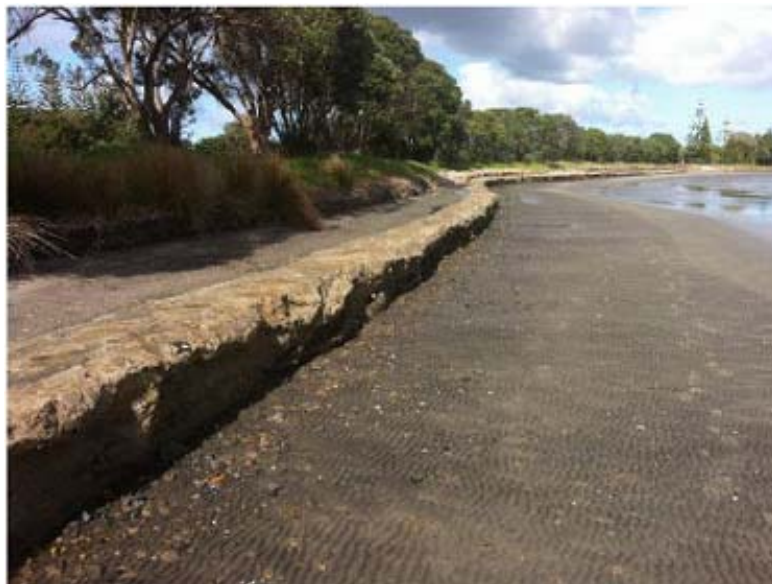
Photograph 3.5.1: Stabilised Sediment Wall forming a public path – Omaha 2012
