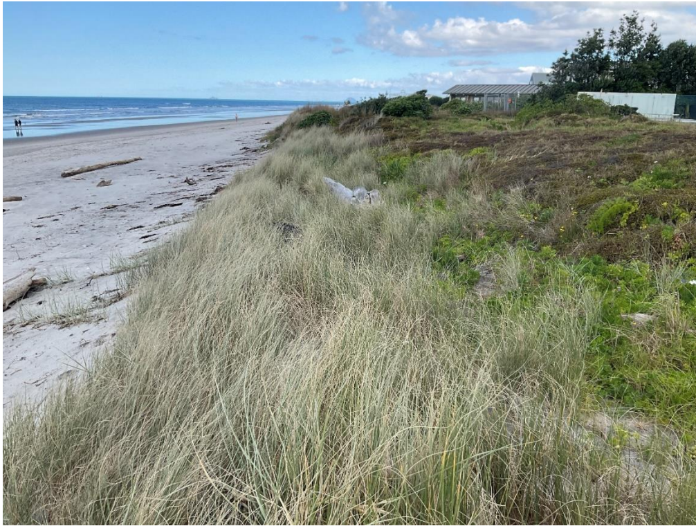
Southern end showing terrace escarpment edge in spinifex and terrace with reasonable pohuehue cover to the right.
