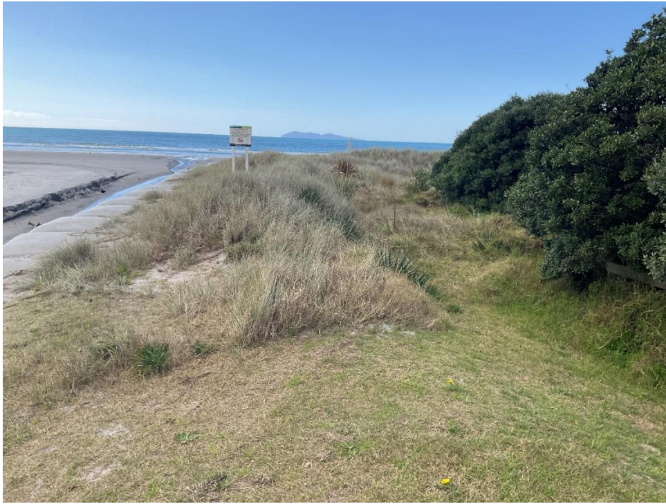
Northern edge from Glen Isla Place access, Three Mile creek and sand bagged edge on left.
