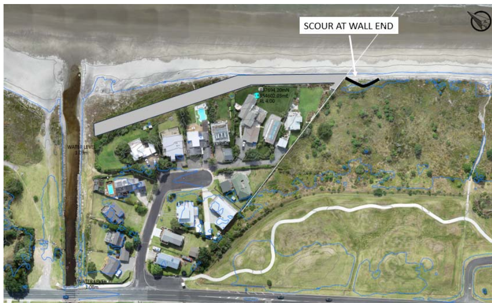
Figure 5.3.2c: Potential scour at southern wall end
