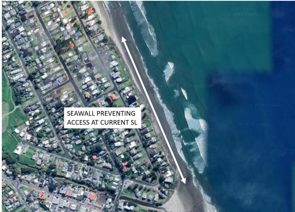
Figure 5.3.4b: Seawall at Shaw Road – water at wall
