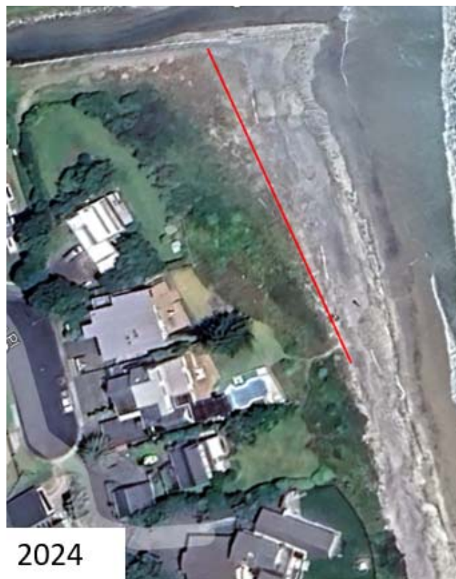
Figure 3.4c: Dune line post groyne construction
