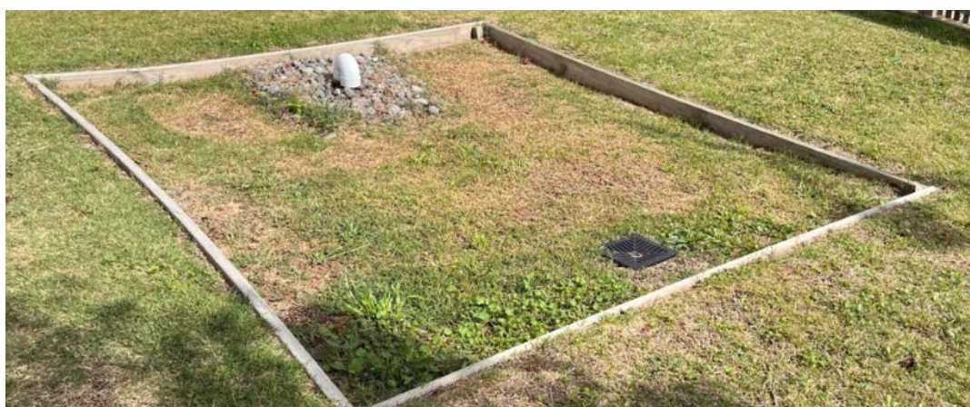
Figure 7: non-compliant raingarden with no vegetation
