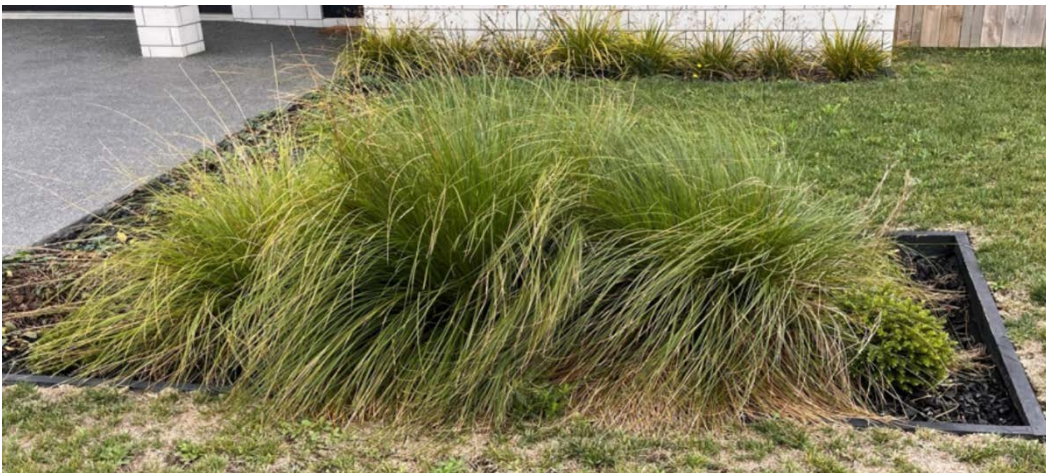
Figure 3: Compliant rain garden with good vegetation
