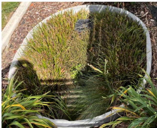
Figure 4: Compliant rain garden in concrete surround
