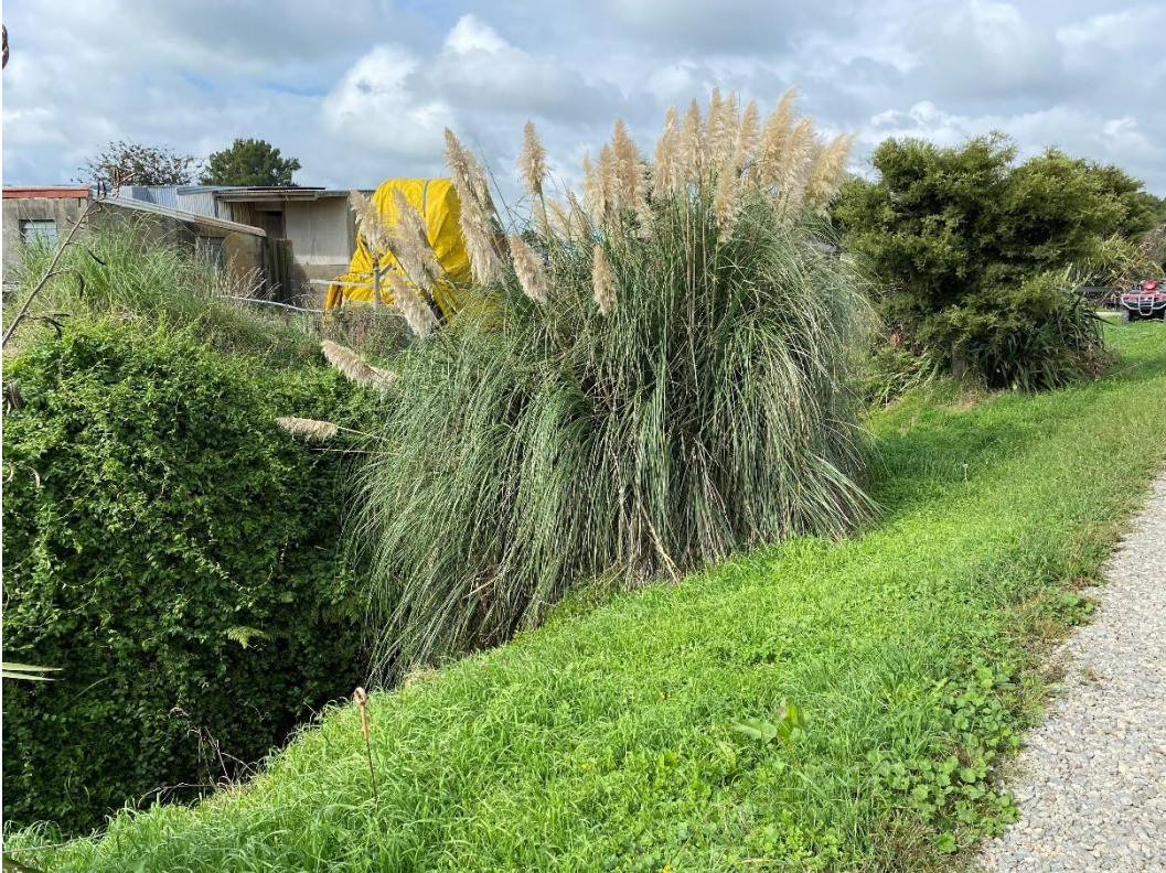
Plate 5: Drain on the western margin of the project area.
