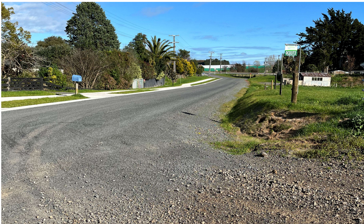
Figure 5.4 Arawa Road looking south from proposed development access
