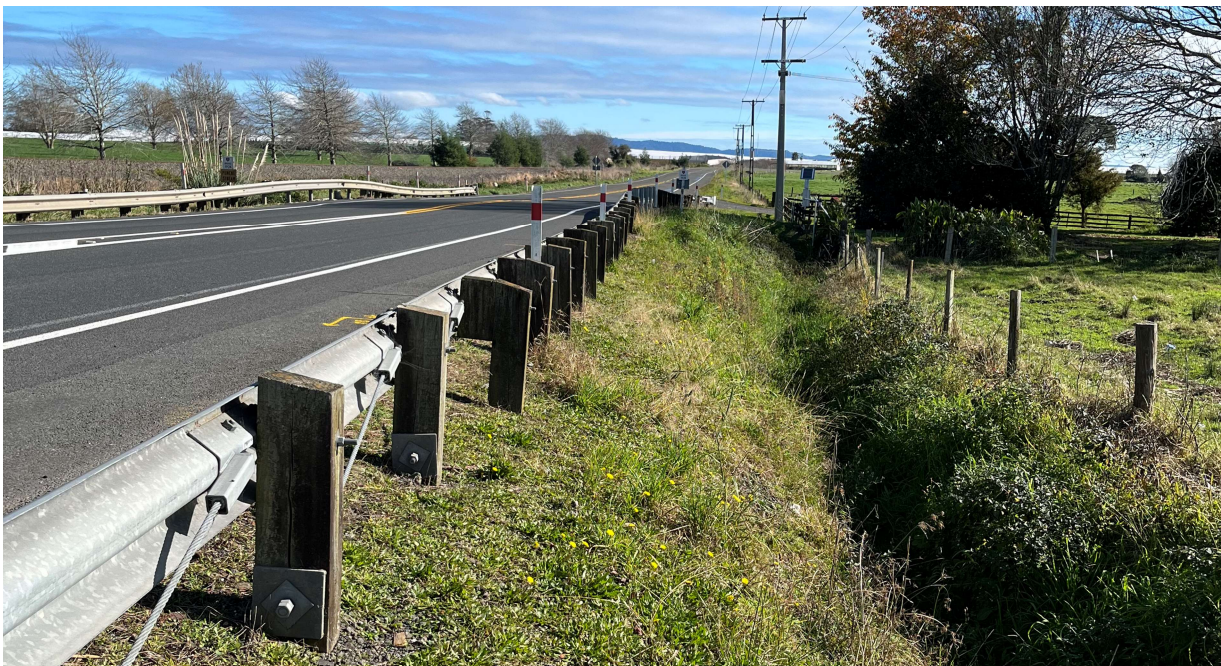
Figure 5.1 Existing roadside barrier which will be relocated adjacent to the power poles and swale
