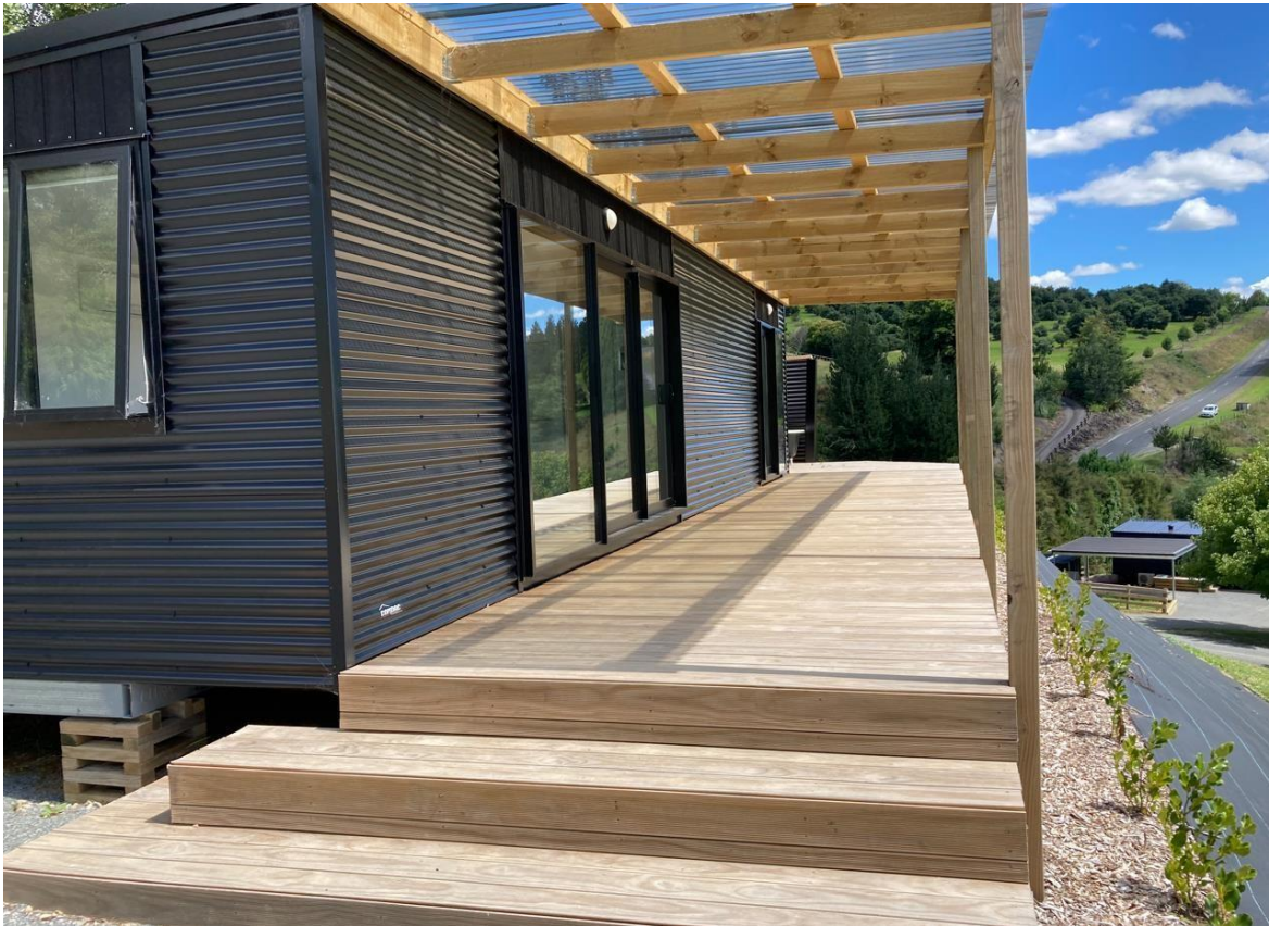
Example of an attached structure (veranda roof)
