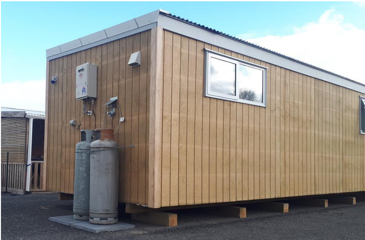
Example of a unit that is not attached to a trailer allowing it to be moved with relative ease.
