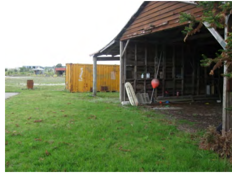
Above: The closed mill buildings (taken from gate)
