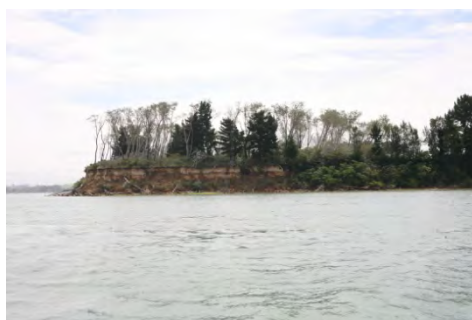
Above: Coastal erosion at Rangiwaewa
