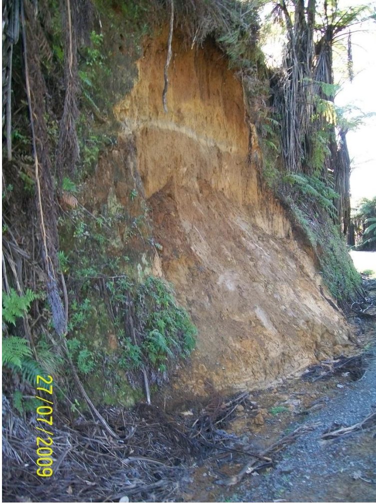
Figure 2: Erosion in the Minden
