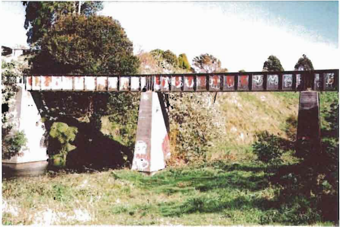
The Rereatukahia Stream Bridge (T14/602) (source: Moore 2002).
