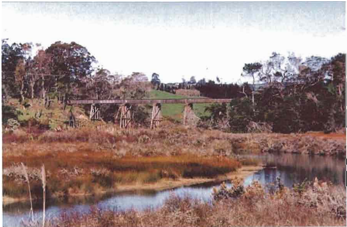
The Wainui River Bridge (U14/3100) (source: Moore 2002).
