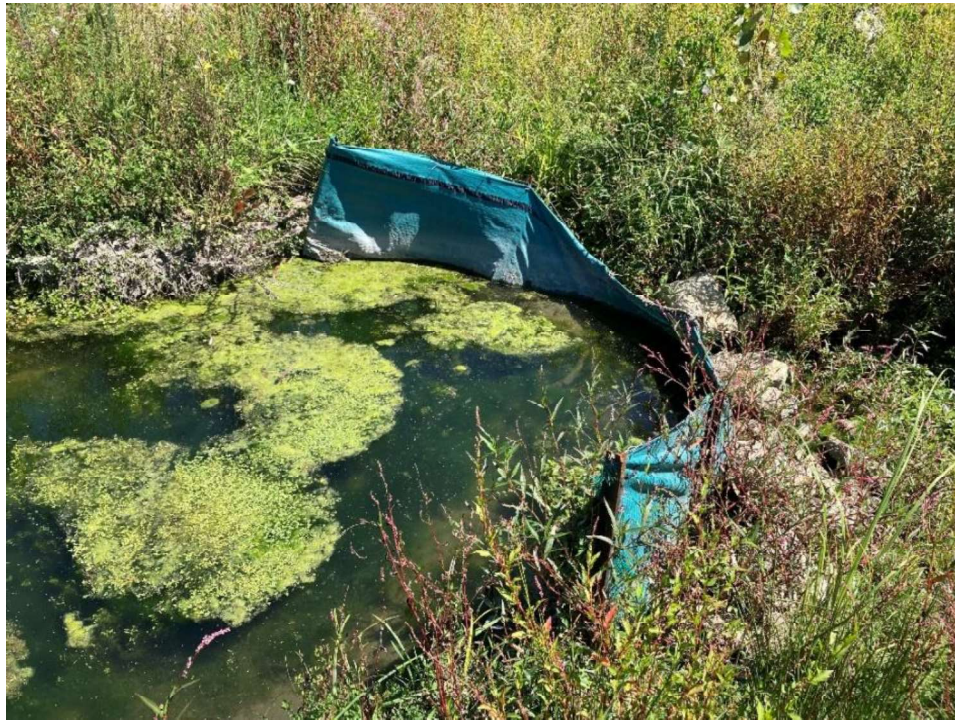
Plate 8: Sediment trap just above the pond which has enabled a small pool of water to bank up behind it. 2 March 2022.
