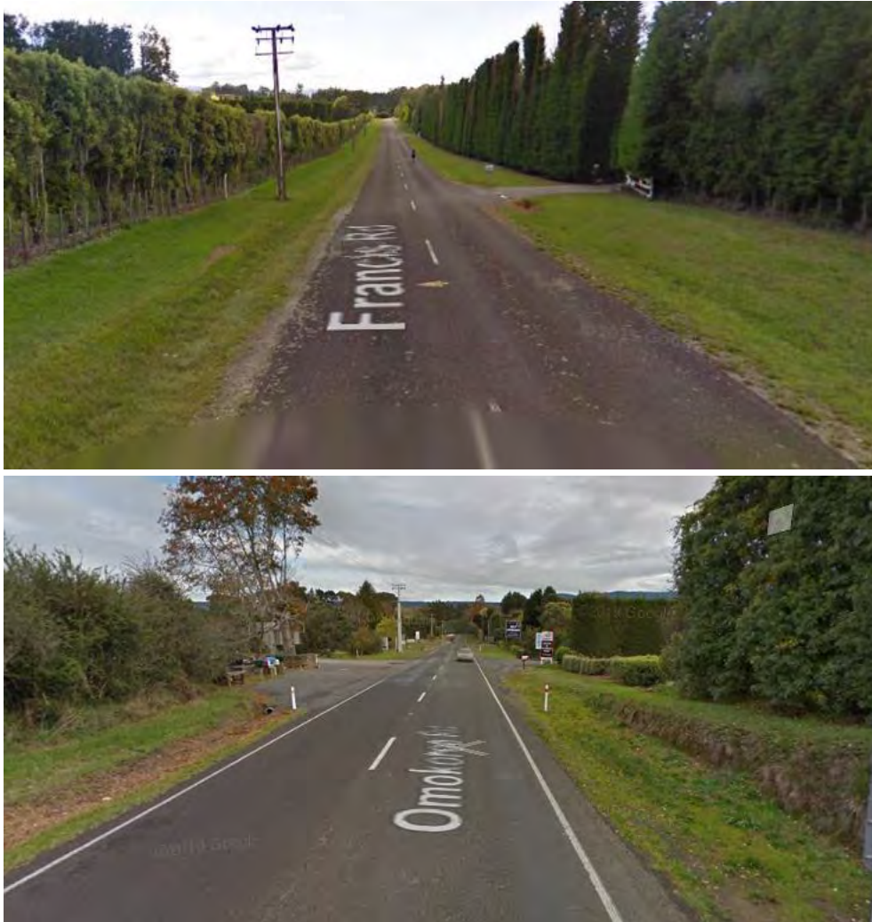
Figure 2-7: Typical carriageway layouts (Francis Rd pictured top, Omokoroa Road pictured bottom. Sourced from Google Street View)
