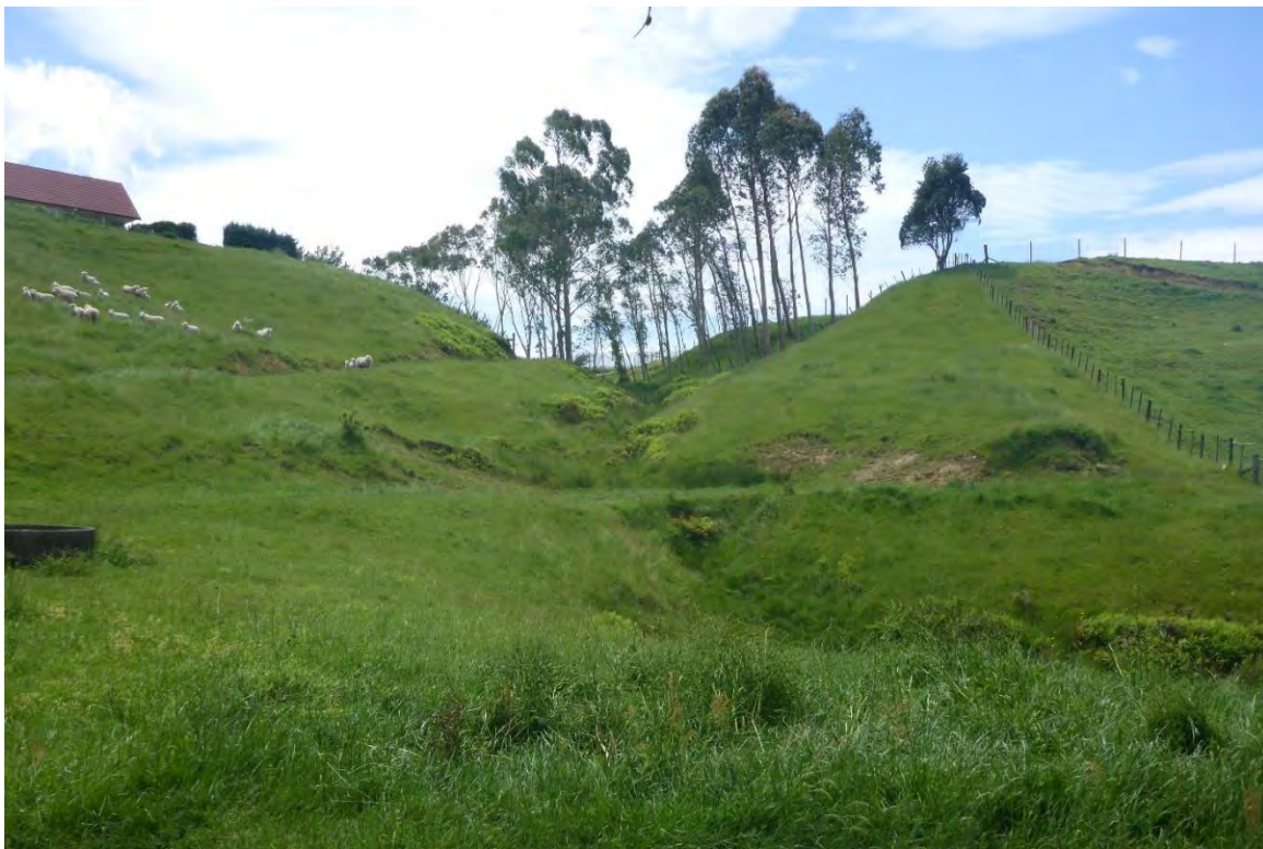
Figure 2-11: Reach Omo_E2 which has the highest erosion susceptibility. Note the steep slope, confined valley floor, access for stock, culvert, and evidence of bank erosion already occurring
