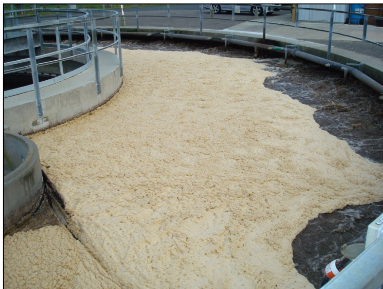
Figure 4 Secondary Treatment Reactors
